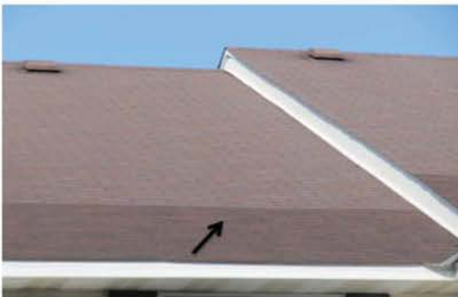
Area of replaced shingles, along eave edge.
