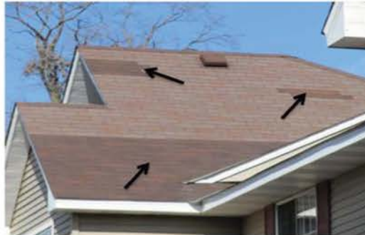
Areas of isolated asphalt shingle replacement.
