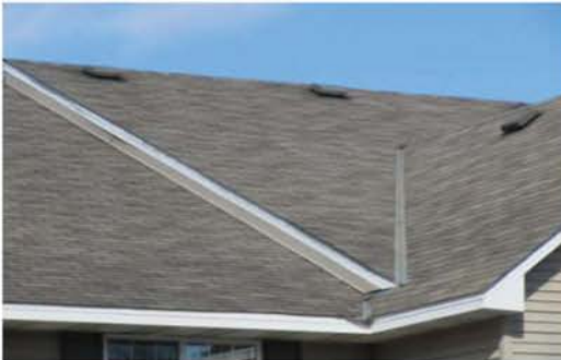
Overview of asphalt shingle roof with valley flashing.
